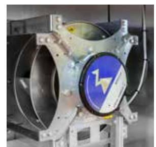
Plug fan with electronically commutated motor
