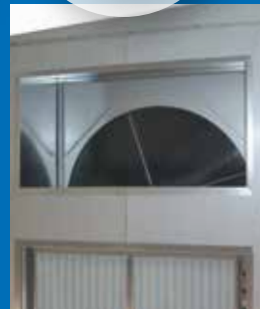
Rotary heat exchanger
