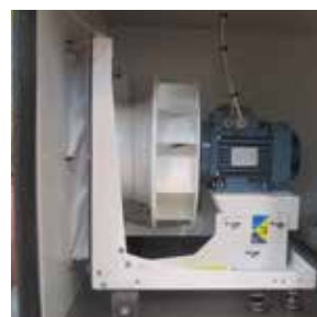
Plug fan with induction motor
